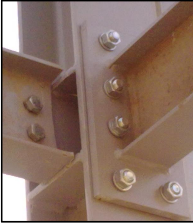
Simple and Moment Connections: Fin Plate and Extended End Plate
