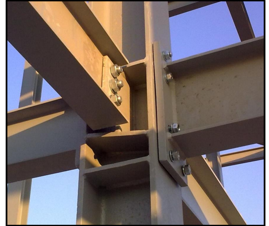
Simple and Moment Connections: Fin Plate and Extended End Plate
